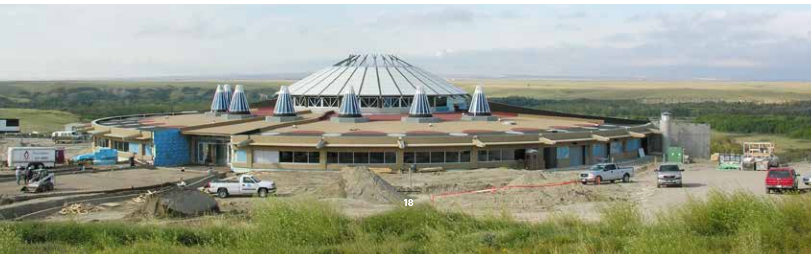
Blackfoot Crossing under final construction, April 2007.
